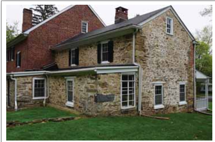
Rear of Hart's original structure.
